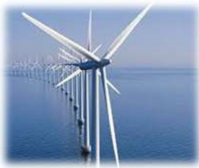
Figure 3. HAWT wind farm
